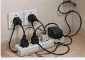
FIRE HAZARDS From overloaded sockets, short circuits, or unattended electrical devices.
